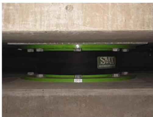
Photo 5: Laminated rubber bearing isolator
